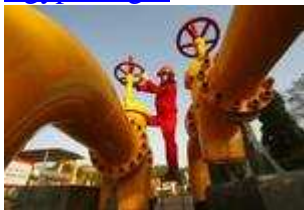
Egyptian gas pipelines - one runs dry
